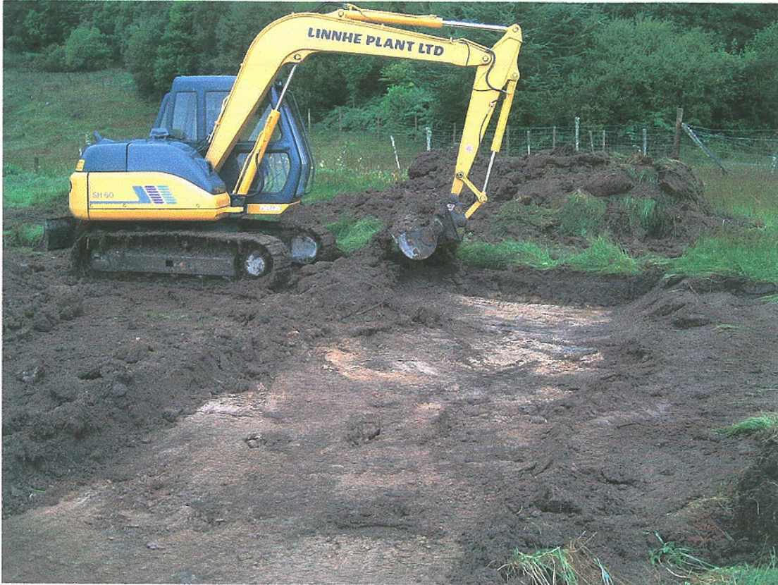
Plate 3. Stripping the car park to a hard surface, from NE.
