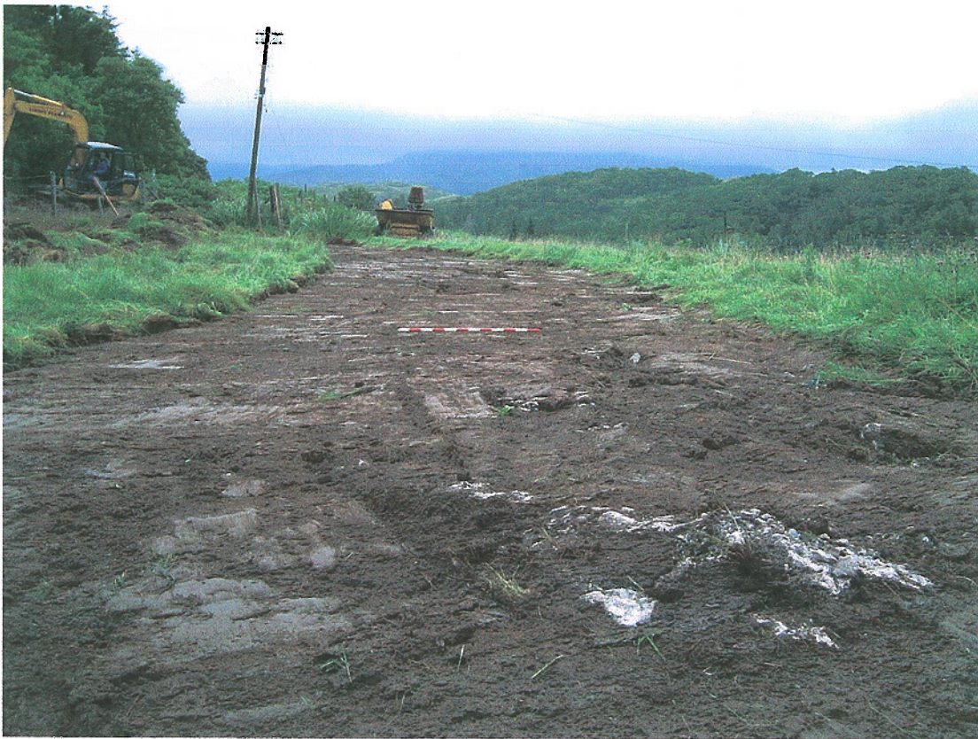
Plate 4. Topsoil stripped from the access road, from SW.
